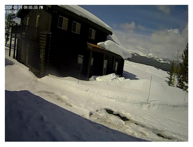
This is a photo of a small roof avalanche near Island Park. Warming temperatures cause water to percolate through the snow which lubricates the sliding surface. Roof avalanches have injured and killed people in the past, just one more thing to worry about. Photo: M.E.
